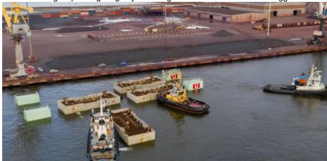
Figur 4-1: Foto: Ugland Construction
