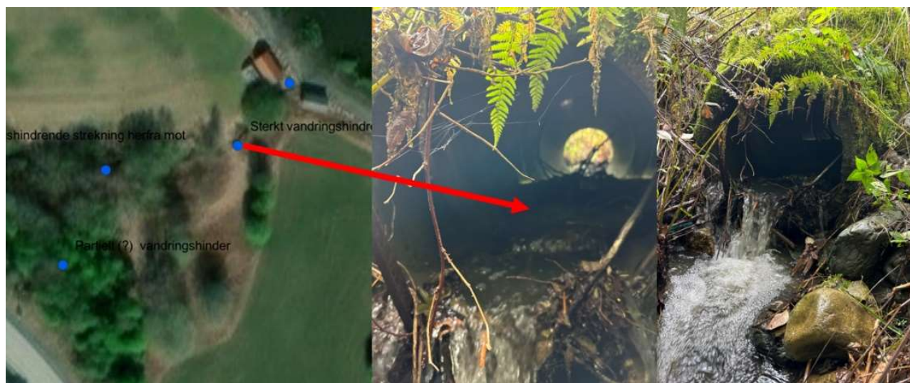
Figur 4-8 Sterkt vandringshindrende kulvert
